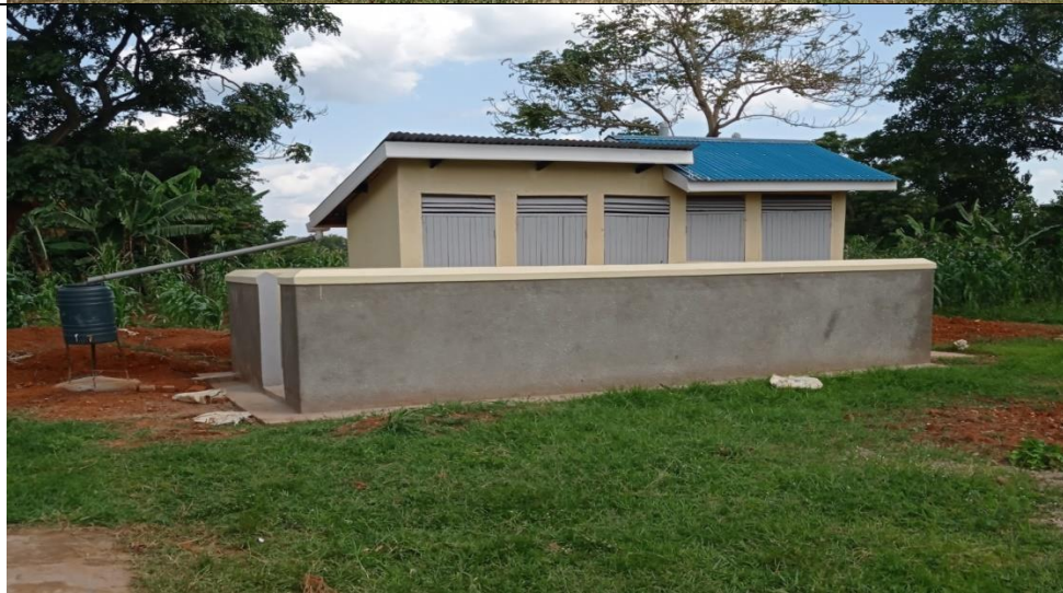
COMPLETED CONSTRUCTION OF 5 STANCE PIT LATRINE AT NABIRAMA P/S IN BUTANSI SUBCOUNTY
