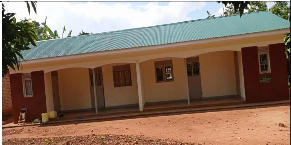
A TWIN STAFF HOUSE CONSTRUCTED AT KASAKA P/S IN BULOPA SUBCOUNTY
