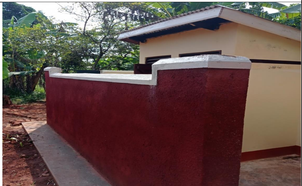
A 2 STANCE PIT LATRINE FOR THE TEACHERS' HOUSE AT KASAKA P/S IN BULOPA SUBCOUNTY
