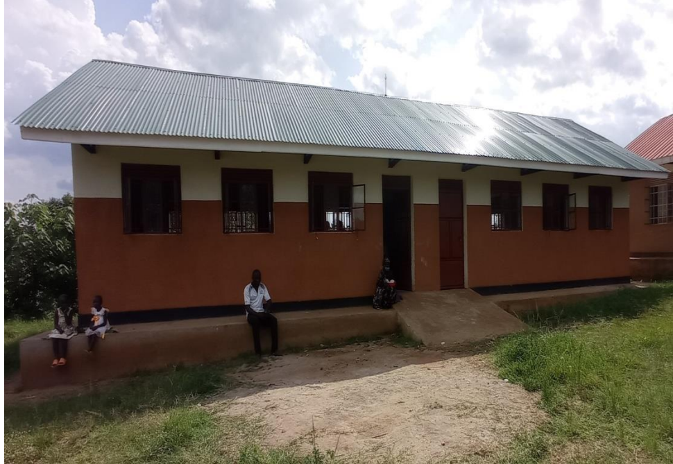
A 2-CLASSROOM BLOCK CONSTRUCTED AT IZANYIRO P/S IN KISOZI SUBCOUNTY
