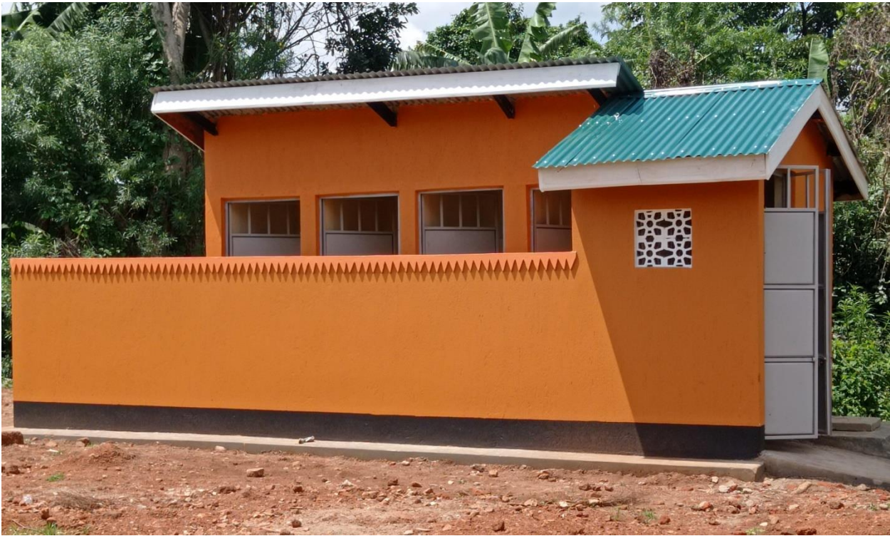
A FIVE STANCE PIT LATRINE CONSTRUCTED AT KIDIKI P/S, NAMWENWA PARISH
